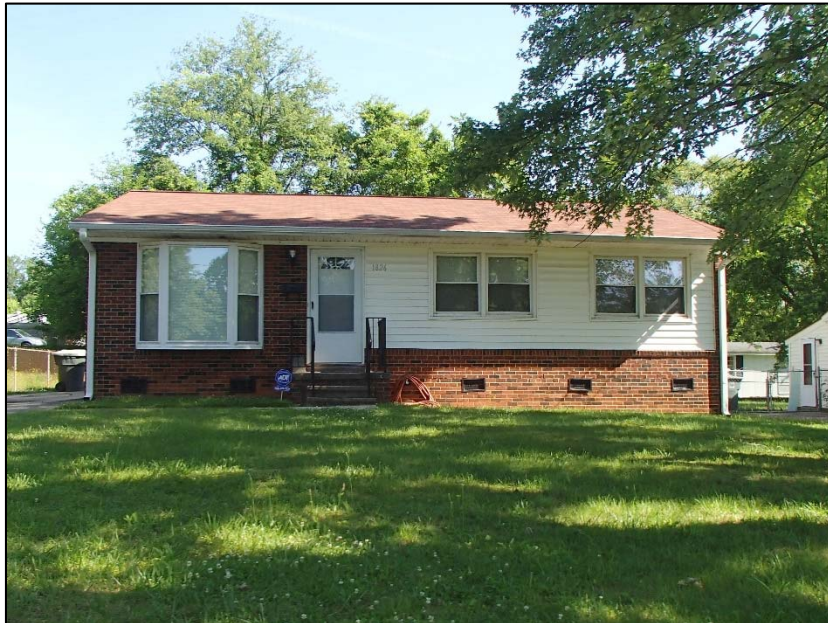
10: Bluford Park house with significant alterations including vinyl siding, replacement windows, new bay window, 1826 Muncey Lane
