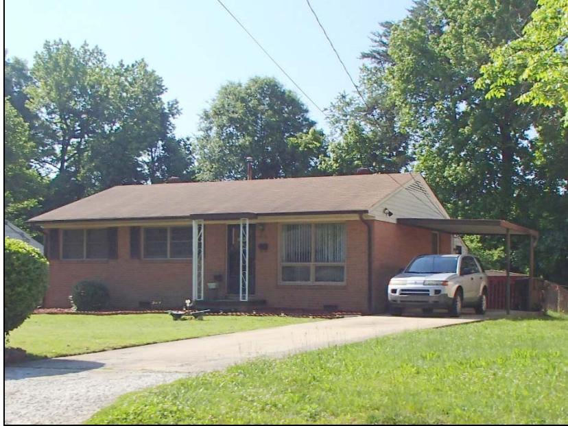
11: Typical Bluford Park house with carport and stoop additions, 1831 Muncey Lane
