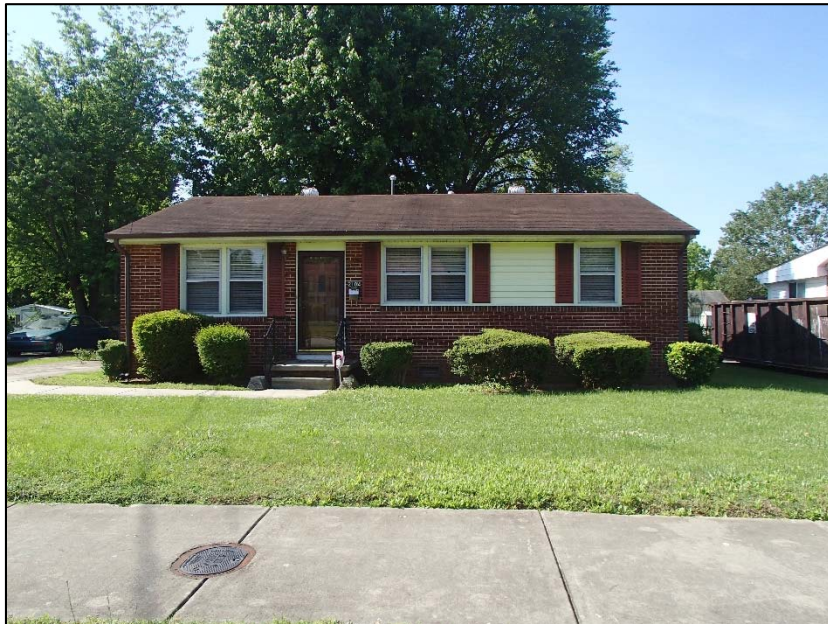
5: Typical Bluford Park house with vinyl siding, 2104 Bothwell Street
