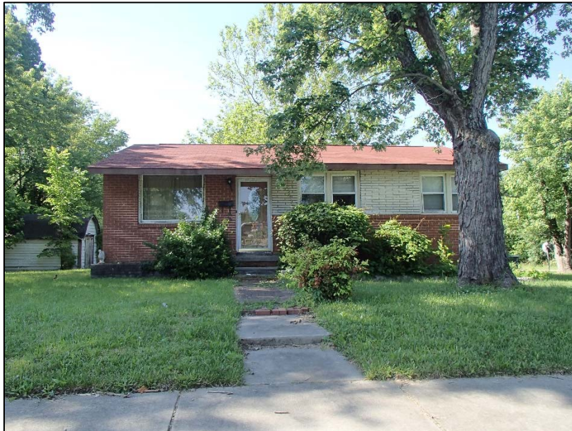
6: Typical Bluford Park house with replacement windows, 2300 Bothwell Street
