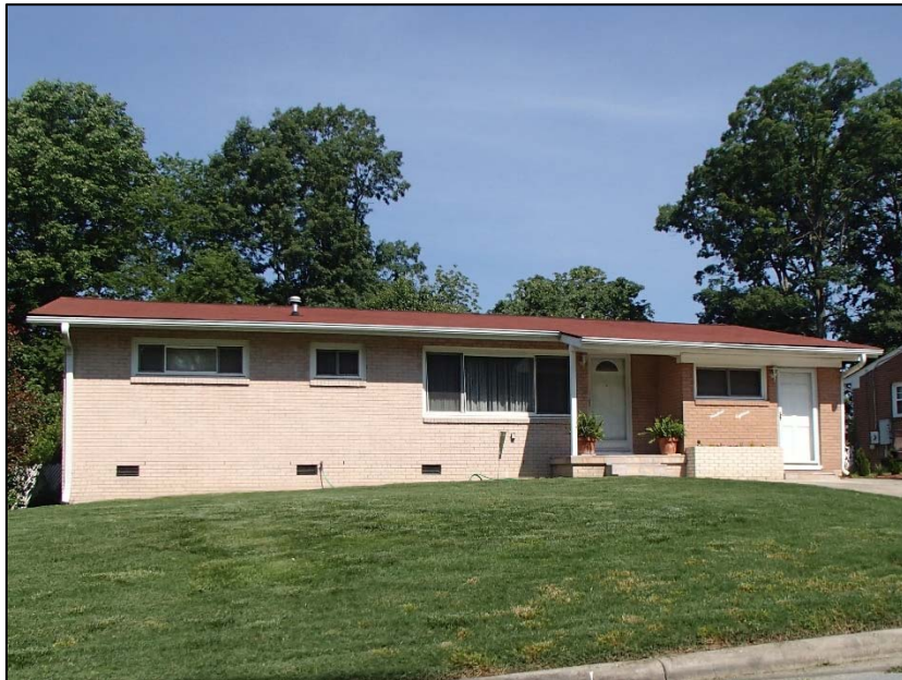
29: Benbow Park house, 1918 Belcrest Drive
