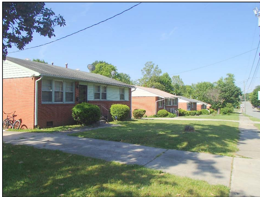
2: 2200 block of Bothwell Street, facing west
