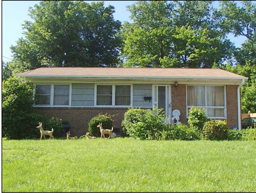
9: Typical Bluford Park house with original asbestos siding and Modernist windows, 2108 Edmund Drive
