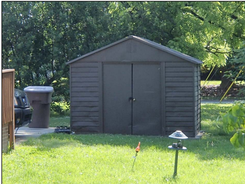
13: Typical Bluford Park prefabricated outbuilding, 1809 Willow Road
